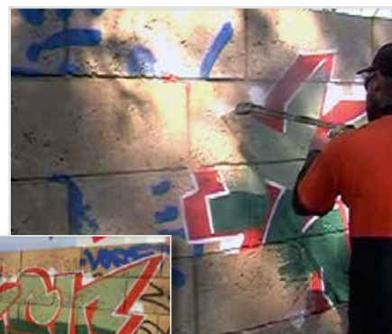
After applying the Coating, it is easy to remove graffiti with hot water alone, or with just one quick application of our removers.
